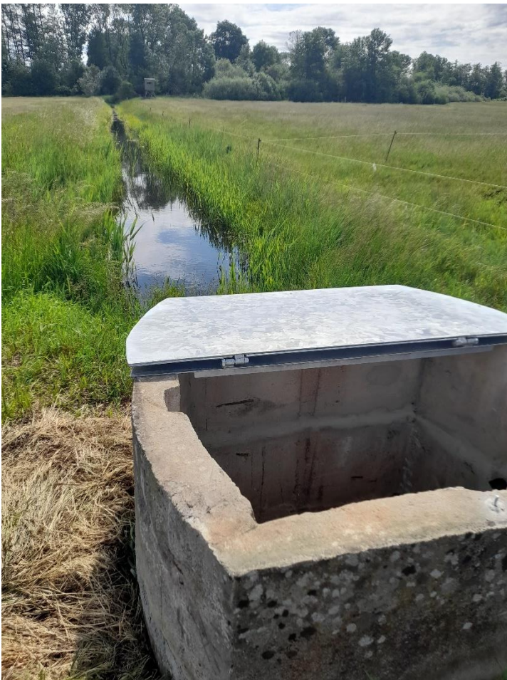
Drainage ditches and a shaft weir between field plots in the Häsener Luch.
