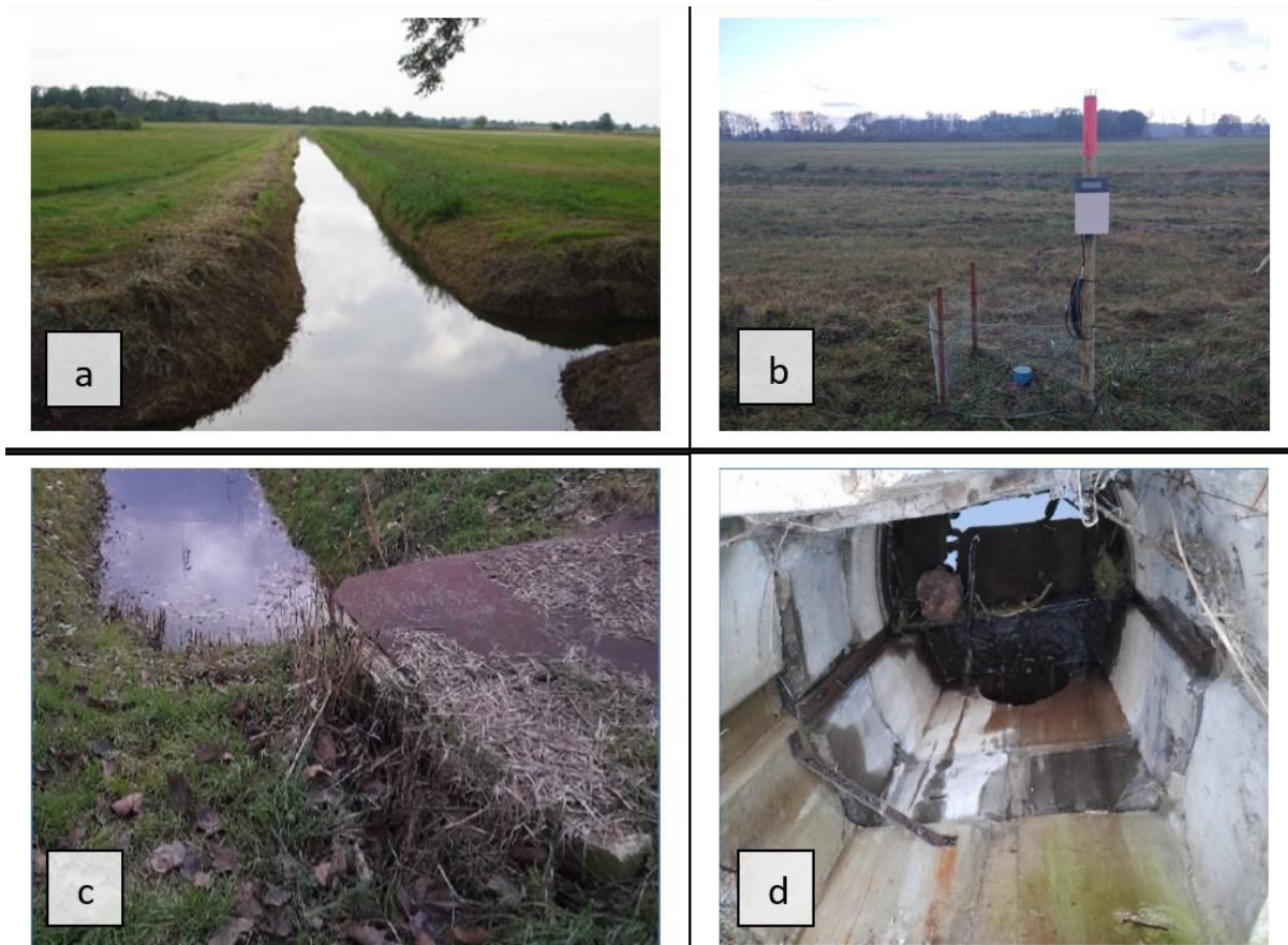
Figure 2.2.2: a) Main drainage channel “Welse-Graben”; b) Installed GW-Pipe on a grassland site; c) Barrage construction exterior and d) interior view
