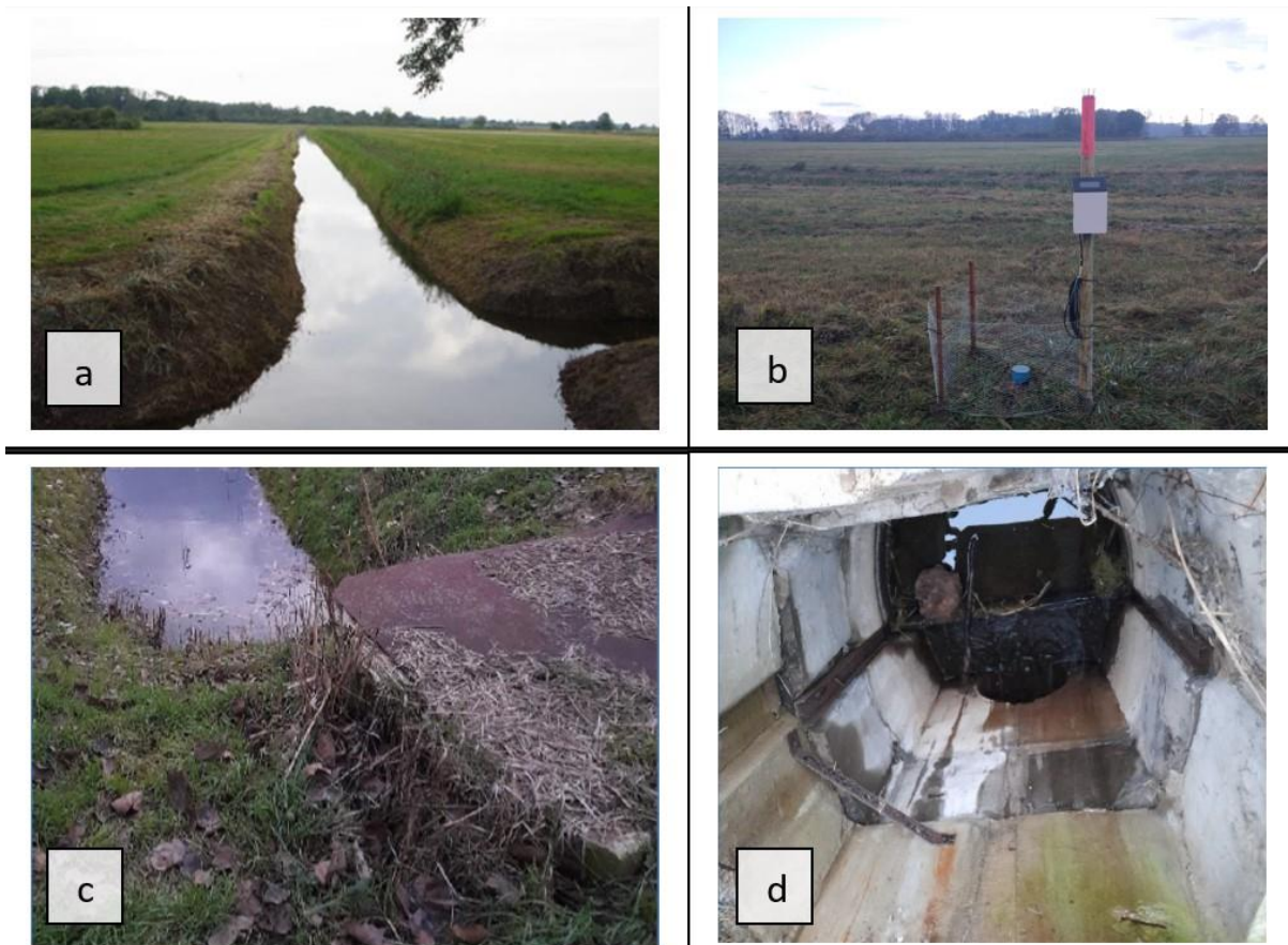
Figure 2.2.2: a) Main drainage channel “Welse-Graben”; b) Installed GW-Pipe on a grassland site; c) Barrage construction exterior and d) interior view
